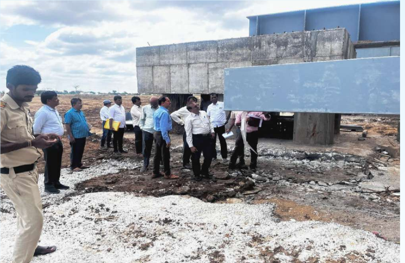
INSPECTION OF HAGARI AQUEDUCT WORKS BY CHARIMAN, TBB
