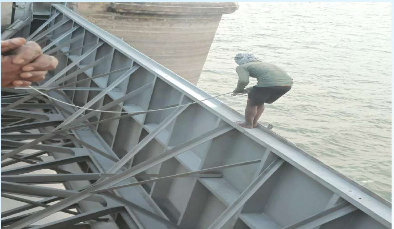
SAND BLASTING AND PAINTING WORK TO THE SPILLWAY GATE NO. 12 TO 22
