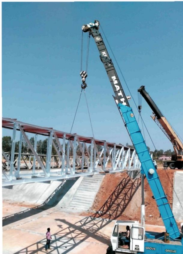
MODERNIZATION WORK STEEL BRIDGE WITHOUT PIERS
