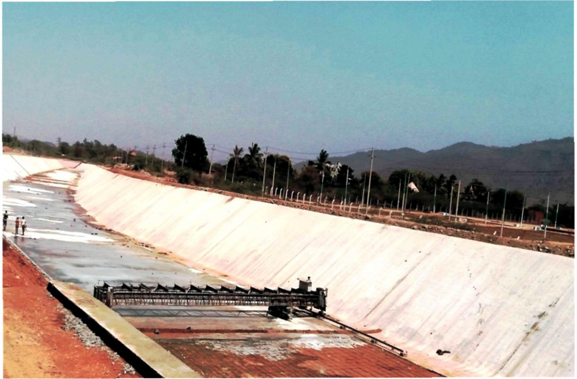
MODERNIZATION WORK AT KM. 6.850. OF RBHLC
