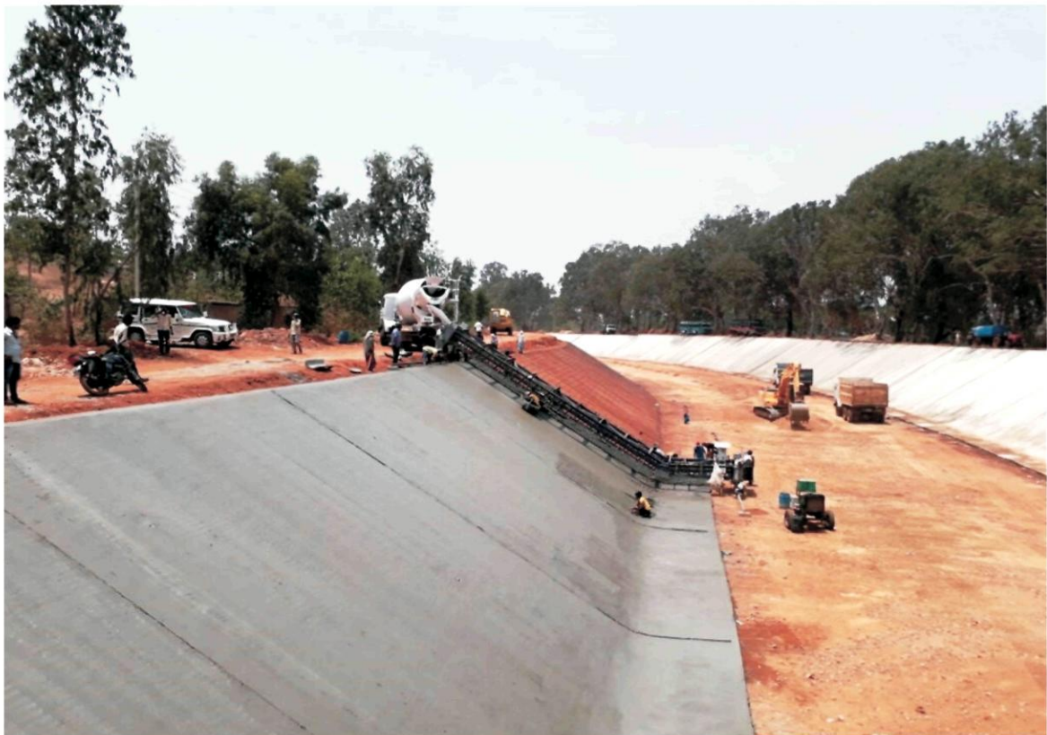
MODERNIZATION WORK AT KM. 2.500 OF RBHLC
