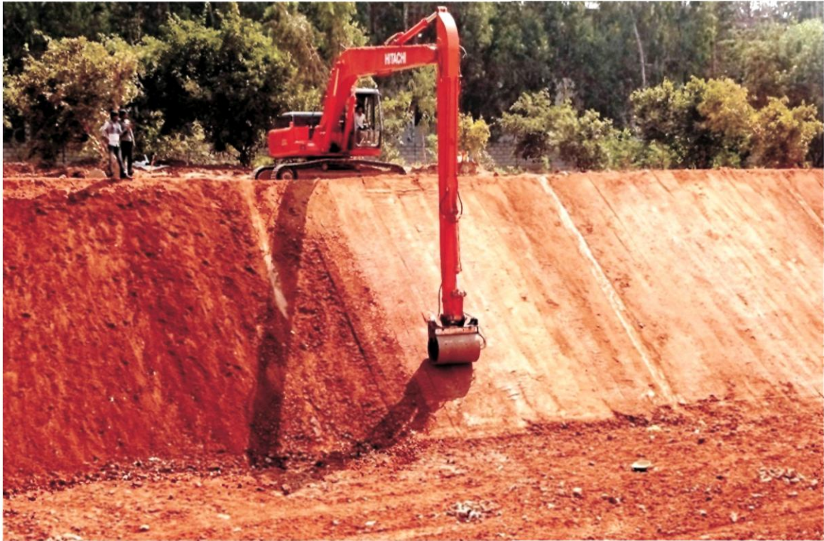
MODERNIZATION WORK AT KM.8.000 OF RBHLC (Slope Compaction with vibrating roller)
