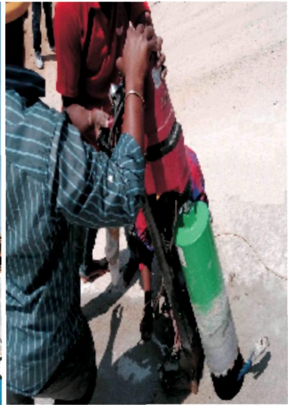
QUALITY CONTROL TEST - CORE TESTING AT 4.400 KM OF RBHLC
