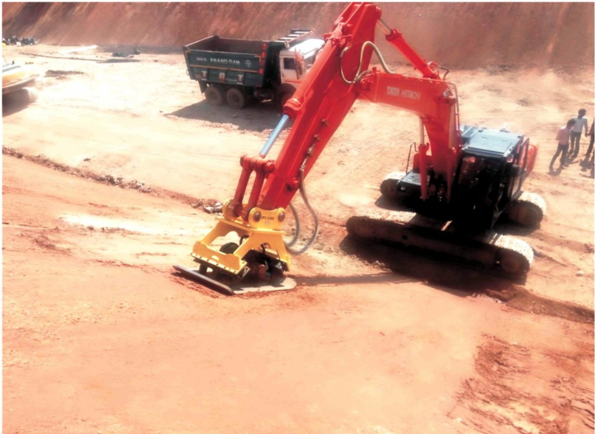
MODERNIZATION WORK AT KM.5.000 OF RBHLC (Compaction with plate vibrator)
