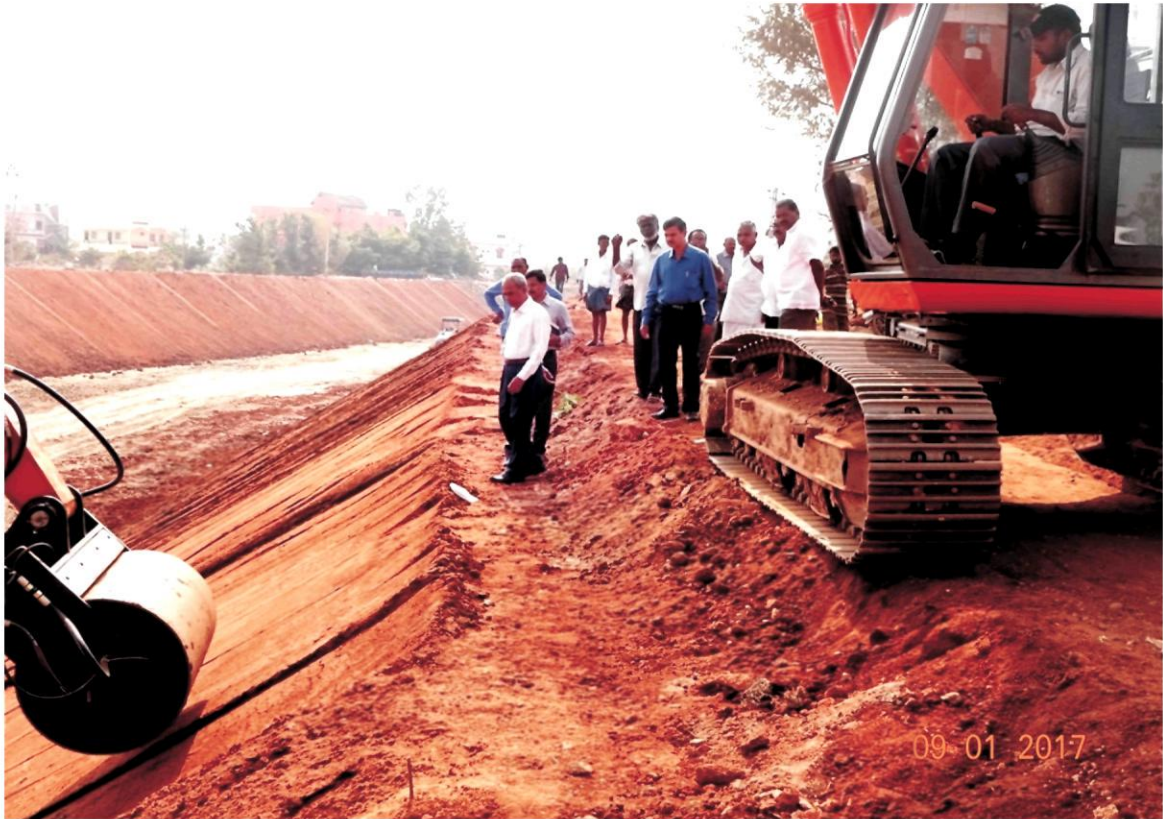
MODERNIZATION WORK AT KM.8.000 OF RBHLC (Slope Compaction with vibrating roller)
